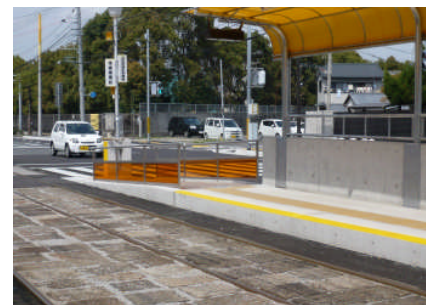
栈橋車庫前電停
